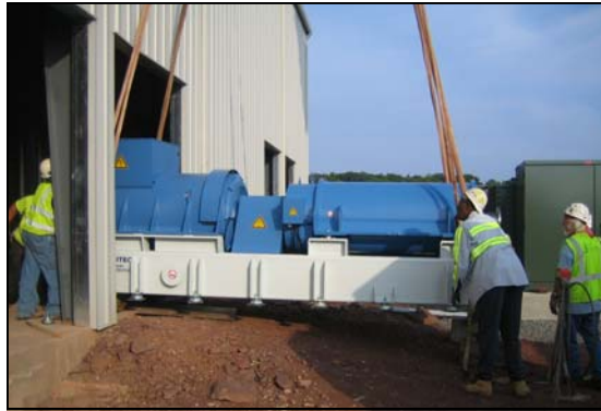
Hitec #2 being swung into place
