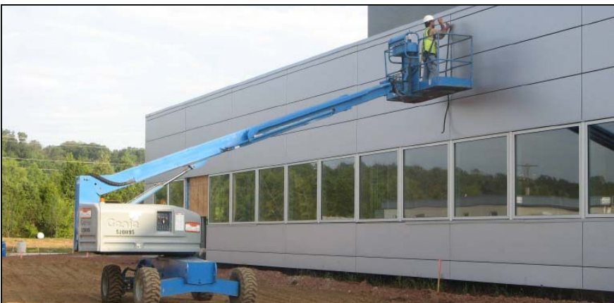
Office skin caulking
